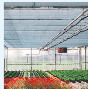
Irrigation boom in a greenhouse with thermic screen . Upper-bar omega shaped due to the heating system.
